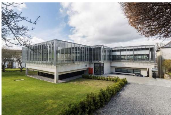
Figure 6: The outside of the refurbished building
